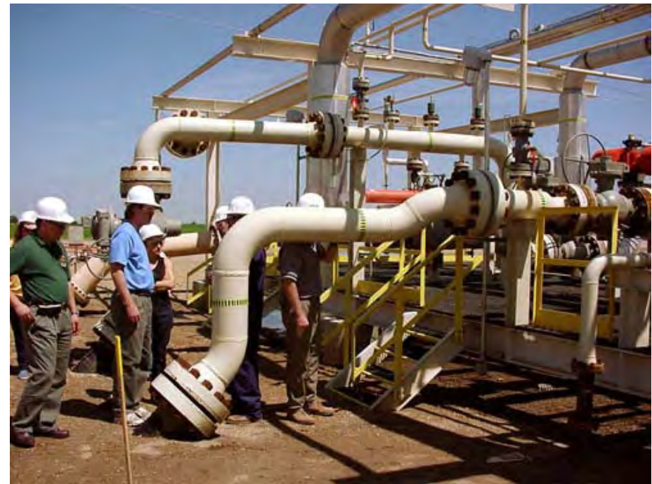
This is where CO 2 arrives after a 320 km pipeline transport from the coal gasification plant with CO 2 capture at Beulah in North Dakota, USA
